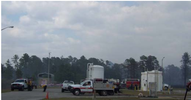
Yankee Lake Water Treatment Fire
